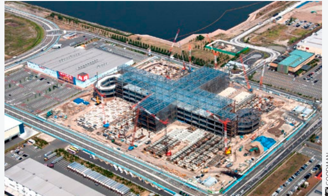
Goodman Sakai is due for completion at the end of March 2014
